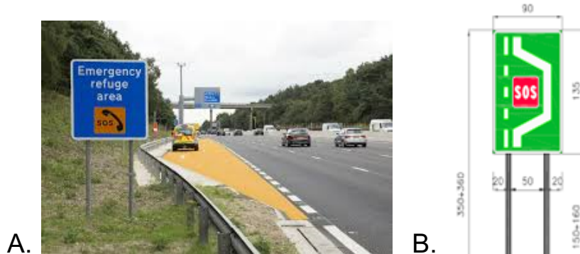
Figure 6. A. UK Motorway refuge area with signage B. Italian signage for refuge area.
